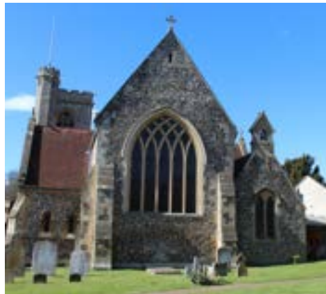
Figure 30 Church of St Mary, eastern elevation
