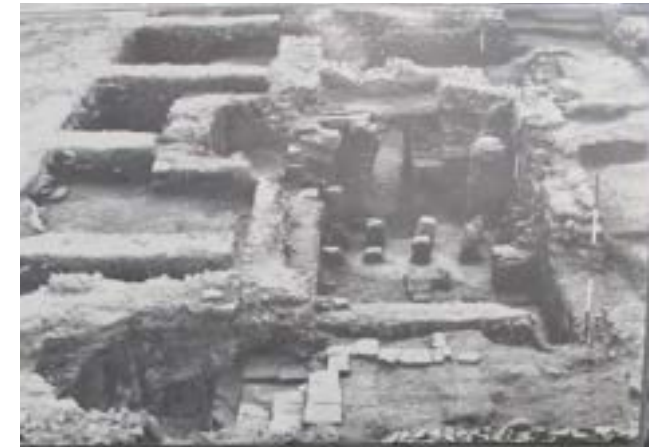
Figure 2 Roman Bath House Excavation (HRO Photo Archive)
