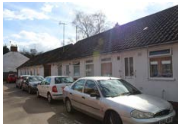
Figure 45 South of Mimram Road
