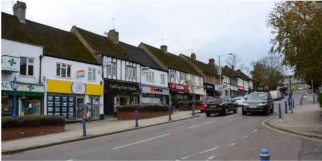
Figure 4.1 Shopfronts along Station Road
